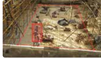
Intrusion Detection of intrusion into dangerous, no-entry zones
